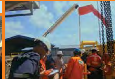
Factory Acceptance Test conducted by clients.
